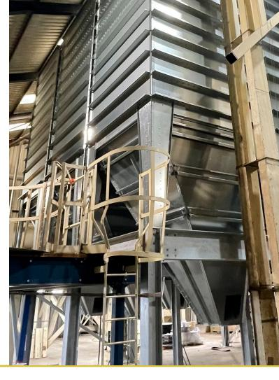
Above all, the customer needed the silos to be completely self-cleaning with no ledges whatsoever to avoid contamination. Therefore, it was crucial to choose bins without inner stiffeners, ensure full discharge, and prevent residues from contaminating future batches.
